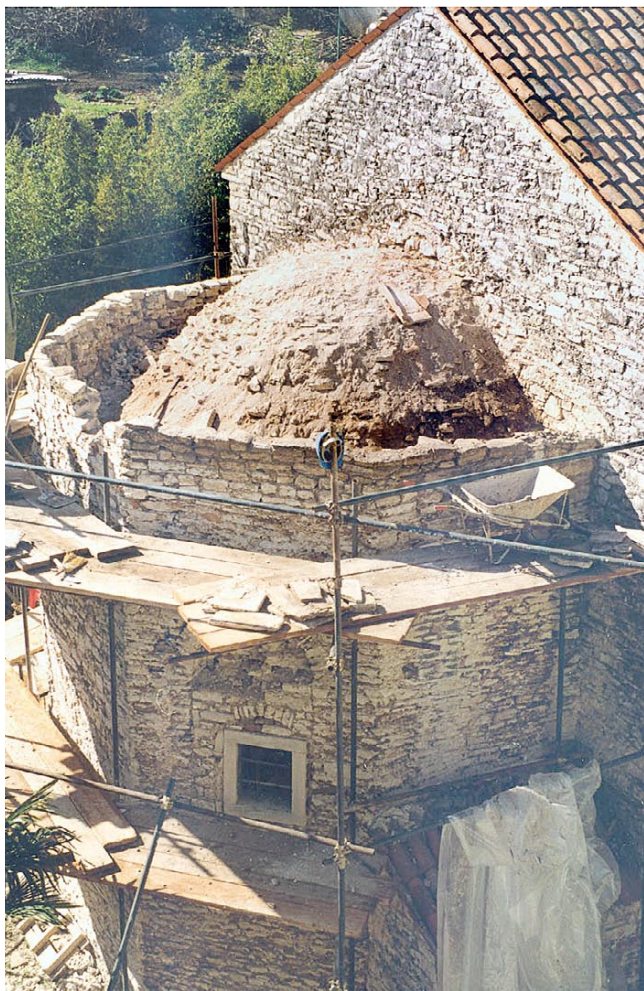
2. Radovi na krovu apside Works on the apse roof
