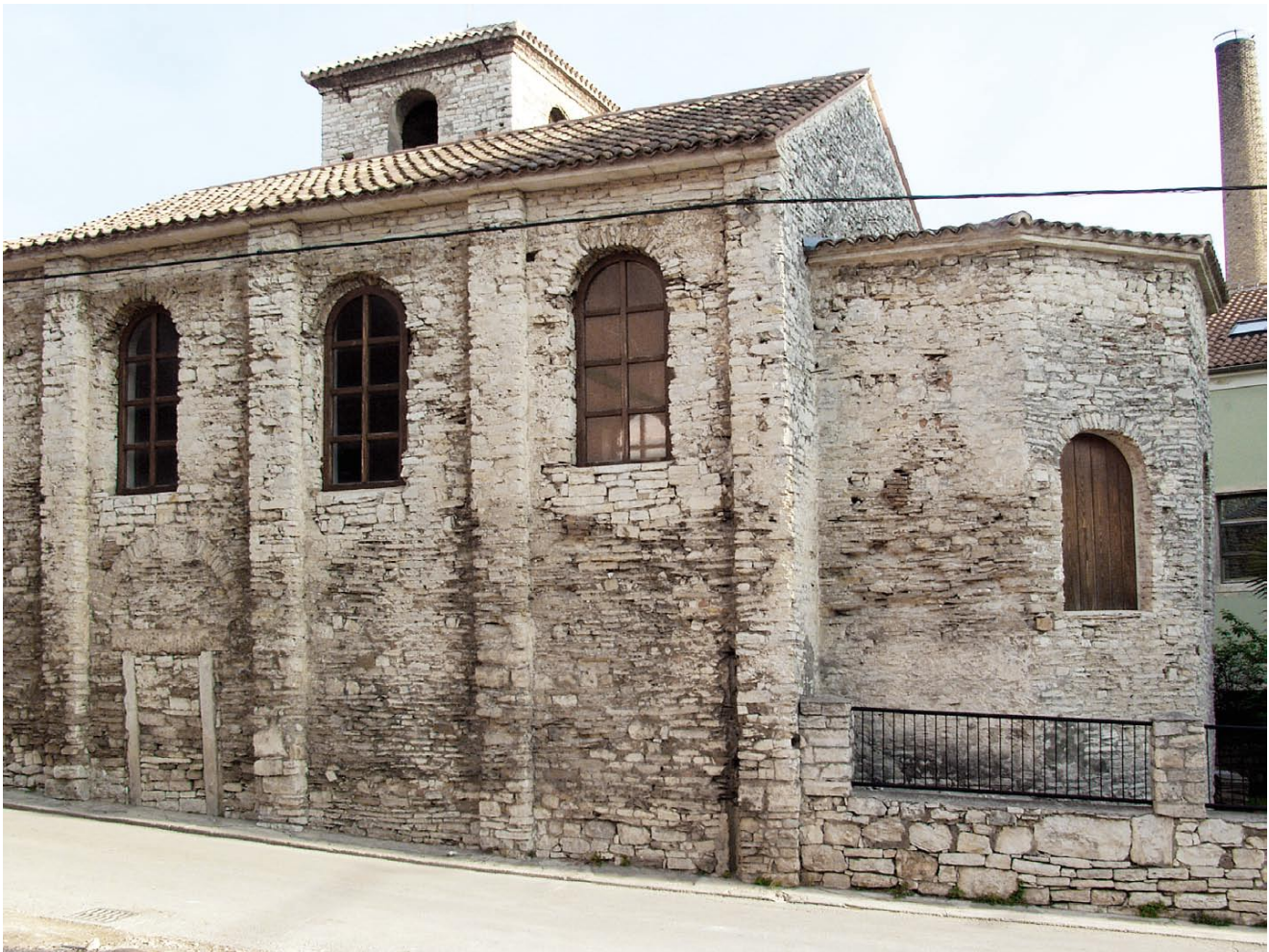
1. Crkva nakon rekonstrukcije pokrova apside i otvaranja prozora (a, b) St Nicholas' after the reconstruction of the apse roof cover and the revealing of windows (a, b)
