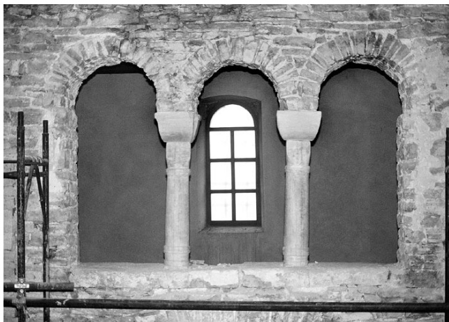
16. Trifora (a, b, c) Trifore window (a, b, c)
