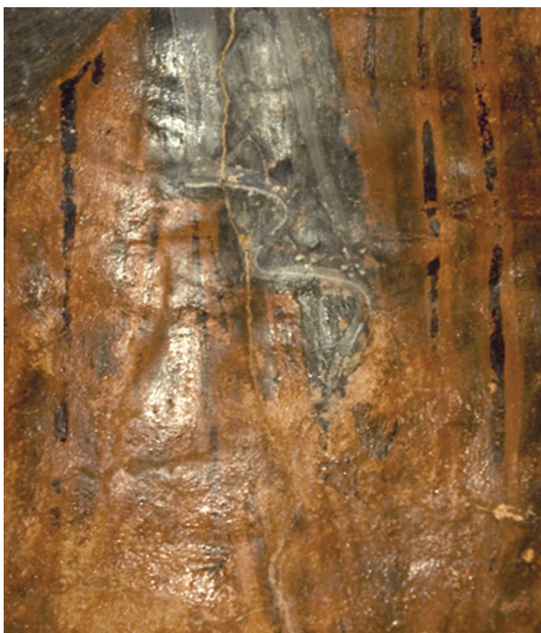
2. Crkva Sv. Ivana, Šilovo selo, detalj oslika u apsidi s kondenznom vlagom na voštanom premazu (fototeka HRZ-a, snimila V. Šulić) Church of St. John, Šilovo Selo, detail of the wall painting in the apse, with humidity condensate on the wax coating (photographic archive of the HRZ, photo by V. Šulić)
