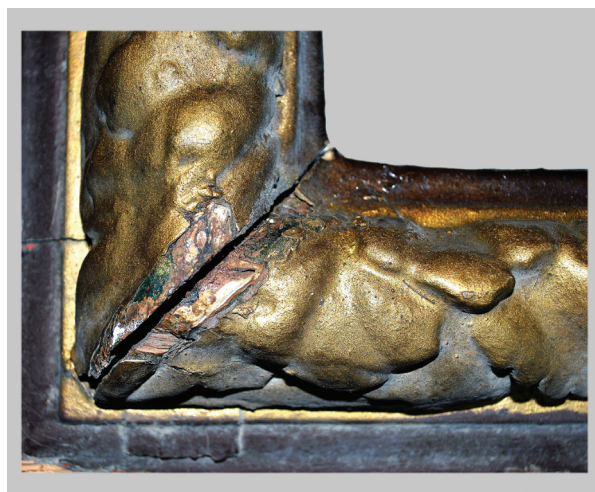
3. Detalj oštećenja kutnog dijela ukrasnog okvira, zatečeno stanje (fototeka HRZ-a, snimila I.N. Unković) Detail of the damaged corner section of the decorative frame, condition before the works (photographic archive of the HRZ, photo by I.N. Unković)
