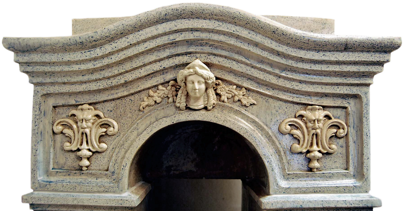
11. Bijela peć, detalj ornamenta nakon nanošenja sloja nove glazure i retuša oštećenja (fototeka HRZ-a) The white stove, detail of an ornament after the application of new glazing and retouching (photographic archive of the HRZ)
