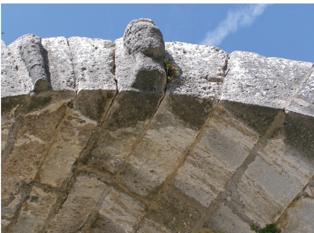
Sl. 8 Crne inkrustacije ispod reljefa glave Herkula Fig. 8 Black incrustations underneath Hercules' head in relief.
