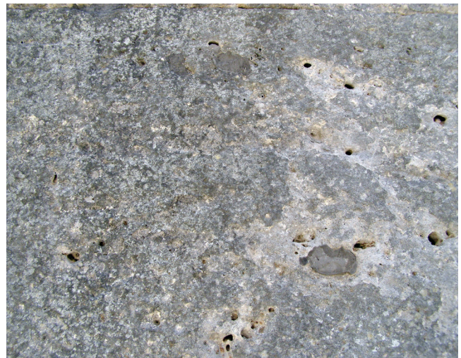
Sl. 11 Primjer velikih alveola zapunjenih cementnim mortom Fig. 11 An example of large alveoli filled with cement mortar.
