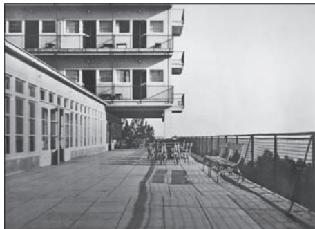
SL. 10. H. BAUER I M. HABERLE: HOTEL KO-OP U ULCINJU, TERASA RESTORANA, 1939.
