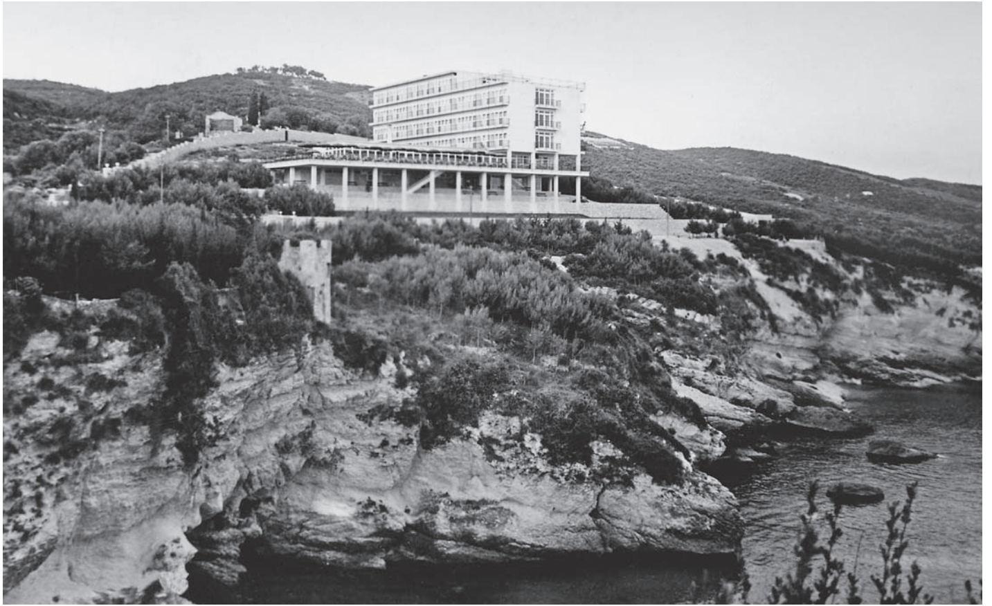
SL. 1. H. BAUER I M. HABERLE: HOTEL KO-OP S BIDIMOVOM KULOM U ULCINJU, 1939., POGLED S MORA FIG. 1. H. BAUER AND M. HABERLE: CO-OP HOTEL WITH BIDIM'S TOWER, ULCINJ, 1939, VIEW FROM THE SEA
