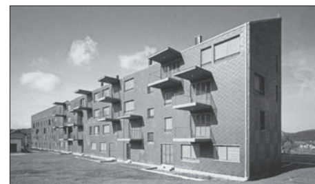
SL 5. DELNICE, STAMBENE ZGRADE, VLADIMIR KASUN I IVICA PLAVEC, 2004. (TLOCRT 1. I 2. KATA / SNIMKA S ISTOKA) FIG. 5. DELNICE, RESIDENTIAL BUILDINGS, VLADIMIR KASUN AND IVICA PLAVEC, 2004 (1 ST AND 2 ND FLOOR PLAN / EAST VIEW)
