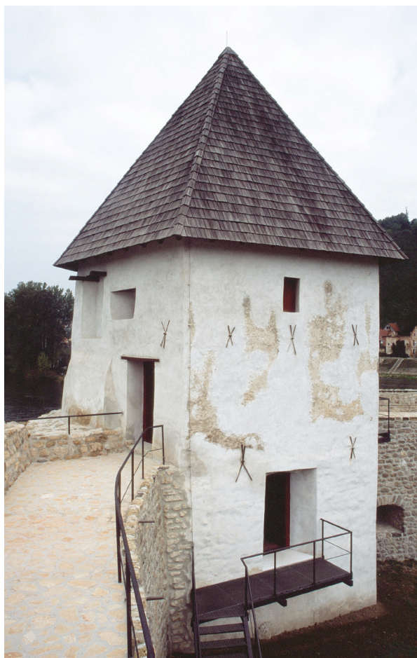
24. Pogled na peterokutnu kulu (2011.) View of the pentagonal tower (2011)
