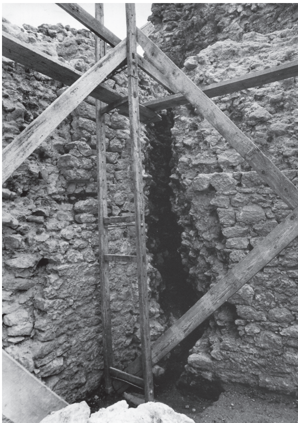
17. Kostajnica, Stari grad, kaverna na spoju istočnog i sjevernog izvornog obrambenog zida Kostajnica, Old Town, cavern at the junction of the east and north original defensive wall
