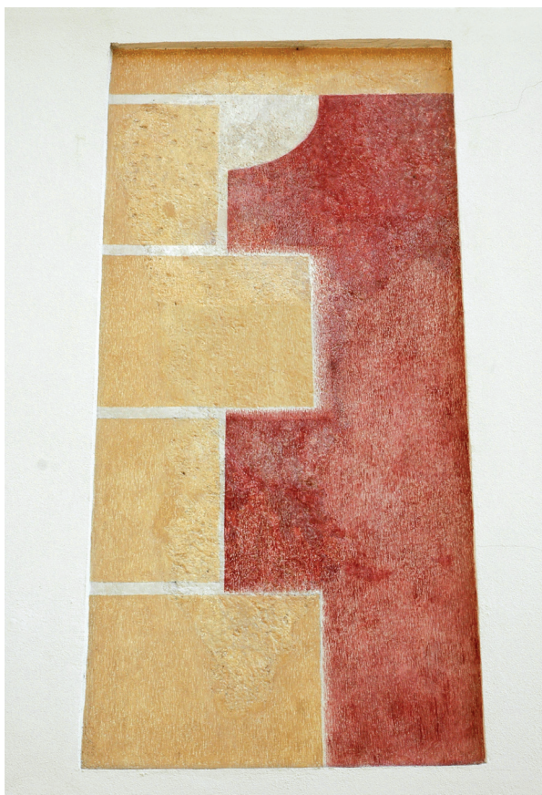
23. Detalj pročelja kuće u Radićevoj 28 u Zagrebu, stanje 2011. (fototeka HRZ-a, snimio I. Srša) A facade detail of the house on 28 Radićeva Street in Zagreb, the 2011 state, (Croatian Conservation Institute Photo Archive, photo by I. Srša)
