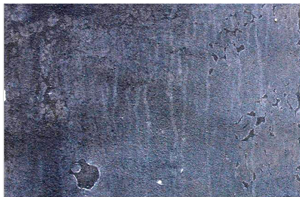
19. Detalj industrijske boje na istočnom pročelju Palaisa, Veliki Tabor, stanje 2011. godine. (fototeka HRZ-a, snimio I. Srša) Detail of industrial paint on the eastern façade of the palace, Veliki Tabor, 2011, (Croatian Conservation Institute Photo Archive, photo by I. Srša)
