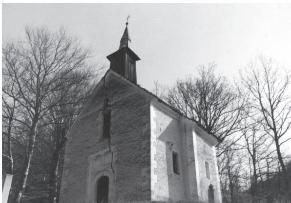
5. Pakra, grobljanska kapela Sv. Nikole, pogled na glavno i južno pročelje (fototeka Ministarstva kulture, snimio N. Vranić, 1957 god.) Pakra, St. Nicholas Cemetery Chapel, view of the southern facade and the main facade with the vertical crack (Photo Archive of the Ministry of Culture, photo by N. Vranić, 1957)
