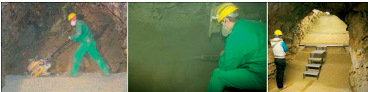
Figure 8 In-situ backfill demonstration at the Josef underground facility.
