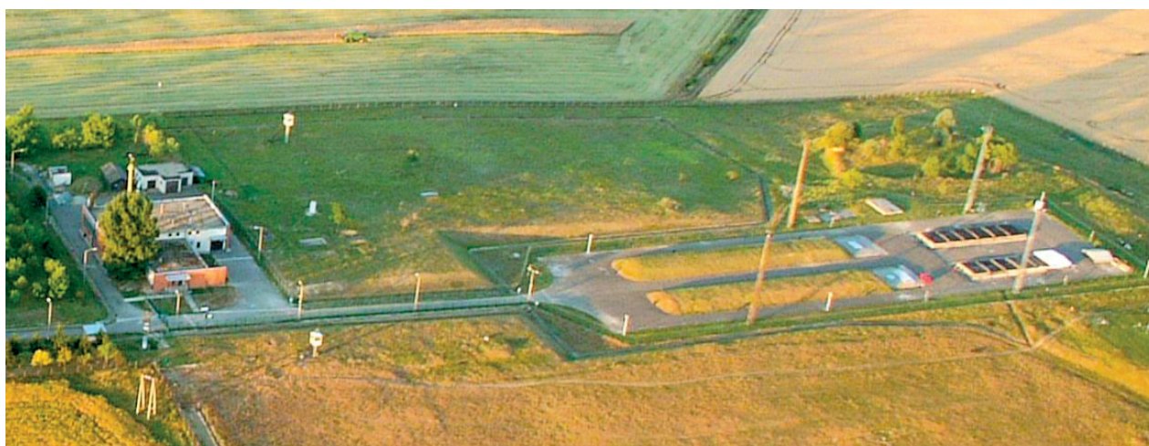
Figure 2. Aerial view of the RWTF. On the left: technological building, on the right the disposal area: two soil covered “A” type vault rows and two without soil cover. “C” type vaults and the steel tubes for SSRS are situated between the soil covered and uncovered rows.
