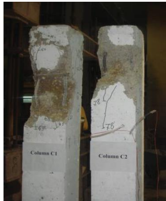
Figure 5. Characteristic damage of columns subjected to axial force. Columns damaged in the upper zone because that part of the column was made from poor concrete (Rabi M.)
