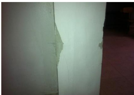
Figure 2. Repair of column damage caused by long-term exploitation
