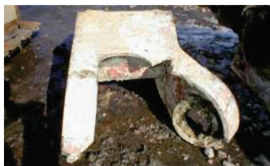
Figure 2 Typical failure of the TWB structure
