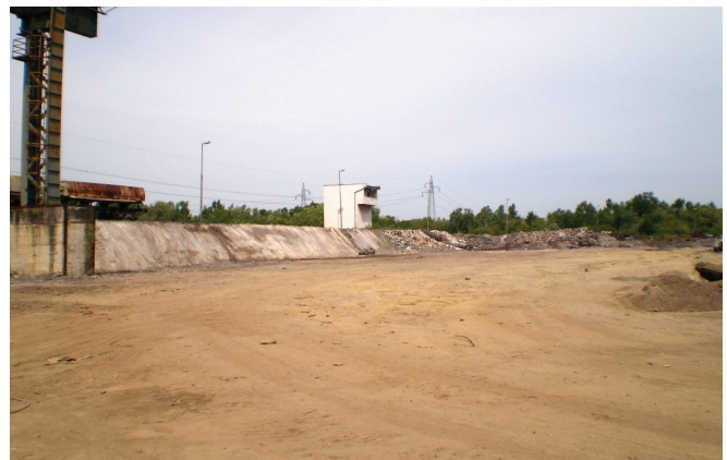
Fig. 2 – Landfill after cleaning and removal of waste
