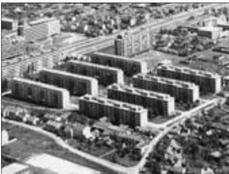
FIG. 5 VLADIMIR POTOČNJAK, STJEPAN GOMBOŠ, VIKTOR HEČIMOVIĆ: EIGHT APARTMENT BLOCKS, 1947/48 (GAJE ALAGE 1-8, FRANA BOŠNJAKOVIĆA 1-8, IVANA STOŽIRA 1-8 AND FAUSTA VRANČICA 1-8)
