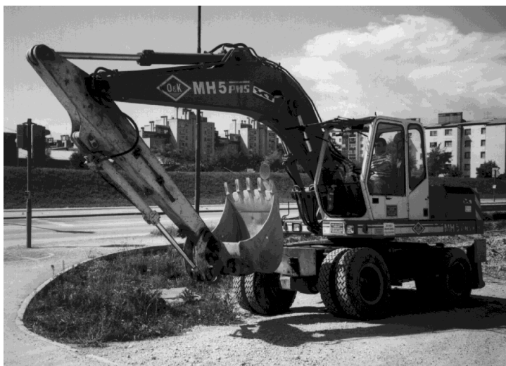
Figure 2: Dredger O&K MH5 PMS
