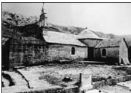
FIG. 7 VIEW OF THE REINFORCED CONCRETE PORCH AND THE CHURCH PRIOR TO 1985 RENOVATION
