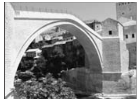
SL. 3. POGLED NA MOST S JUGA, NAKON OBNOVE FIG. 3 VIEW OF THE BRIDGE FROM THE SOUTH, POST-RECONSTRUCTION PERIOD
