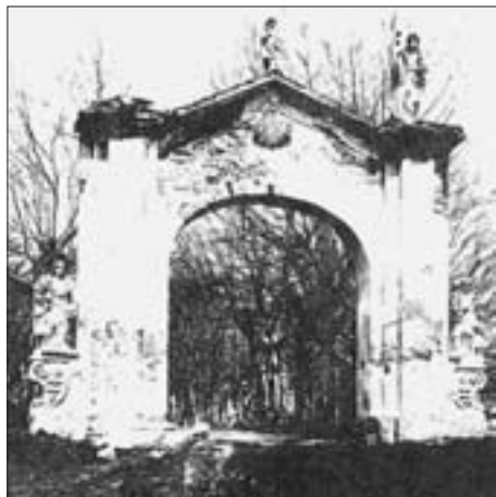
FIG. 3 IVAN STANDL: PORTAL OF THE SANCTUARY AFTER THE 1880 EARTHQUAKE
