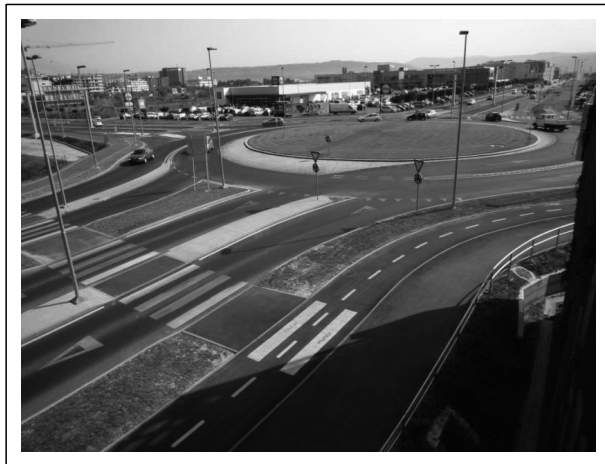
Figure 1 - Turbo roundabout; City of Koper, Slovenia
