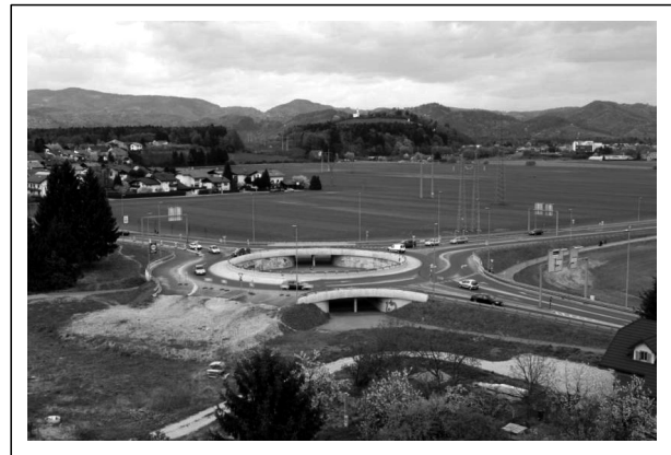
Figure 3 - Typical Slovenian turbo roundabout; City of Maribor
