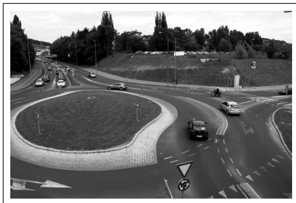
Figure 2 - Physical separation of traffic lanes on a turbo roundabout; City of Maribor, Slovenia
