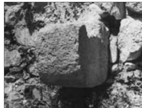
FIG. 4 SUSEDGRAD CASTLE: ONE OF SEVERAL STONE CANTILEVERS NEXT TO THE ENTRANCE WHICH PROBABLY SUPPORTED THE EAVES
