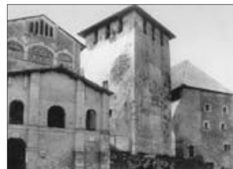
FIG. 9 DEFENSE TOWERS AND PALACES: A (UP) – OZALJ, A DEFENSE TOWER WITH ITS NEWLY-RECONSTRUCTED ROOF STRUCTURE; B (DOWN) – BOSILJEVO, FRANKOPAN'S CASTLE BEFORE ITS RECONSTRUCTION IN THE 19 TH C.: DEFENSE TOWER (IN THE MIDDLE) AND A GREAT PALACE (RIGHT)
