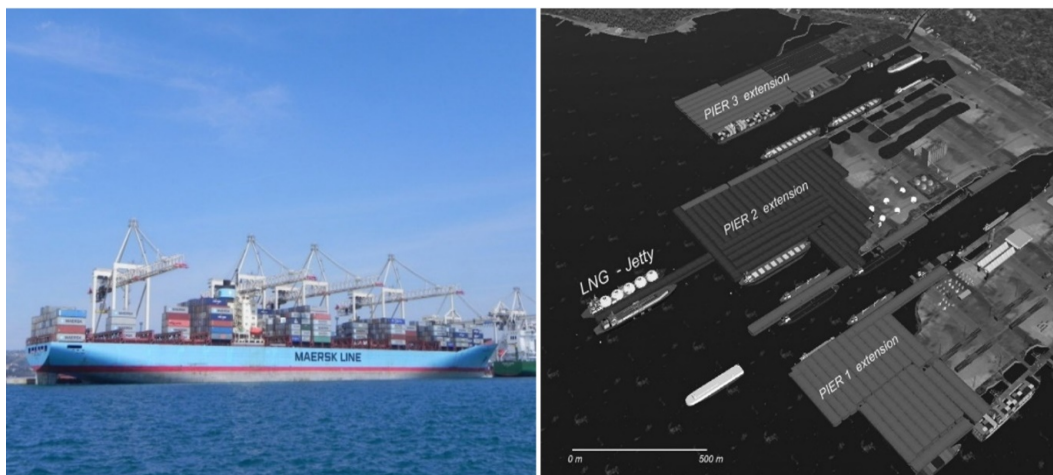
Figure 3 A container vessel on limited draught alongside the existing container terminal, and the extended container terminal
