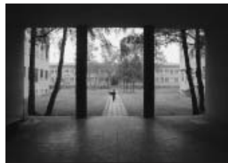
SL. 19. Z. VRKLJAN I N. KUČAN: ZGRADA INSTITUTA I KLINIKA, POGLED IZ PASAŽA TEORETSKO-EKSPERIMENTALNOG SKLOPA FIG. 19 Z. VRKLJAN AND N. KUČAN: INSTITUTE AND CLINIC, VIEW FROM THE PASSAGE OF THE COMPLEX FOR THEORETICAL RESEARCH AND EXPERIMENTAL STUDIES
