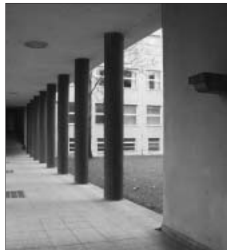
SL. 14. TEORETSKO-EKSPERIMENTALNI SKLOP, SEKVENCA TRIJEMA FIG. 14 COMPLEX FOR THEORETICAL RESEARCH AND EXPERIMENTAL STUDIES; PART OF THE PORTICO
