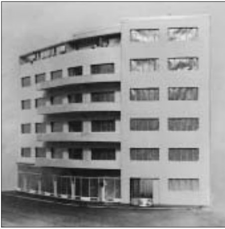
SL. 13. STAMBENO-TRGOVAČKA UGLOVNICA HOFFMANN-SINGER, KRALJA ZVONIMIRA 26 – ŠUBICEVA, 1936.-1937., ING. BOGDAN PETROVIC, MODEL S ULIČNE STRANE FIG. 13 RESIDENTIAL AND COMMERCIAL CORNER BUILDING HOFFMANN-SINGER, KING ZVONIMIR 26 – ŠUBICEVA, 1936-1937, ENG. BOGDAN PETROVIC, MODEL, STREET VIEW
