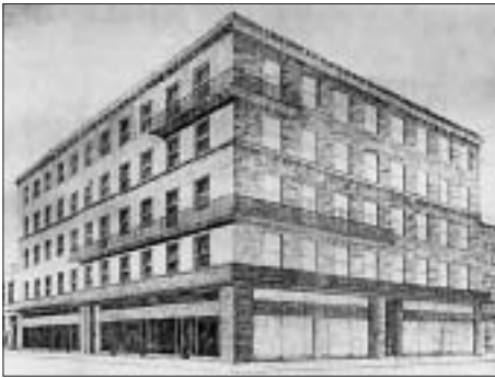
SL. 15. STAMB.-TRGOVAČKA UGLOVNICA BAUM, JURISIĆEVA 30 – TRG HRV. VELIKANA, 1928.-1929., BELA AUER, ZA POSLOVNICU IGNJAT FISCHER, IZVELO GP ING. CERNJAK I NEUMANN FIG. 15 RESIDENTIAL AND COMMERCIAL CORNER BUILDING BAUM, JURISIĆEVA 30 – HRVATSKIH VELIKANA SQUARE, 1928-1929, BELA AUER, BRANCH OFFICE IGNJAT FISCHER, BUILT BY CONSTRUCTION COMPANY, ENG. CERNJAK AND NEUMANN
