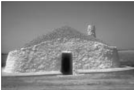
FIG. 1 A MAINTAINED BOMBO IS WHITEWASHED. THE GRAVELLED ROOF OF SOME BUILDINGS IS ALSO WHITEWASHED. SL. 1. ODRŽAVANI BOMBO JE OKREČEN. POŠLJUNČANI KROV NEKIH ZDANJA TAKODER JE OKREČEN.
