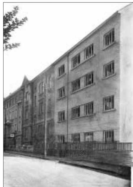
SL. 13. FOTOMONTAŽA PROCELJA UGRAĐENE NAJAMNE KUĆE ŠNIDARIĆ, ZAGREB, PETROVA 28, 1939., ATTR. JOSIP LIEBICH, URUDŽBENI PROJEKT ZA GRAĐEVNU DOZVOLU FIG. 13 ŠNIDARIĆ BUILT-IN APARTMENT HOUSE - FAÇADE; PHOTOMONTAGE, ZAGREB, PETROVA 28, 1939, ATTR. JOSIP LIEBICH, MAIN DESIGN FOR THE BUILDING PERMIT
