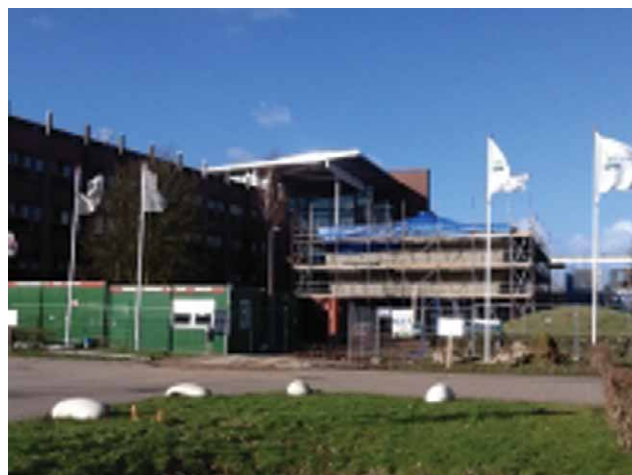
Slika 2. Nova zgrada muzeja tla-Wageningen. Figure 2. New soil museum building-Wageningen
