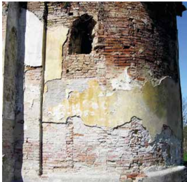
20 Crkva Bogorodice, Koprivna, 13. st. – otklesane opeke lezene polukružnoga svetišta, (foto: D. Pešut, fototeka restauratorske radionice Oslik – Čepin) Church of the Holy Mother, Koprivna, 13 th c., dressed brick of the lesene of the semi-circular sanctuary (photo: D. Pešut, photo archives of the restoration workshop Oslik Čepin)
