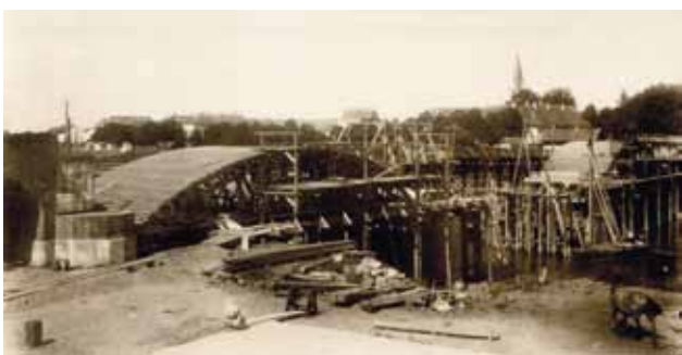
8 Izgradnja mosta na Kupi (GMS, inv. 137 F) Construction of the bridge on the Kupa River (GMS, inv. 137 F)
