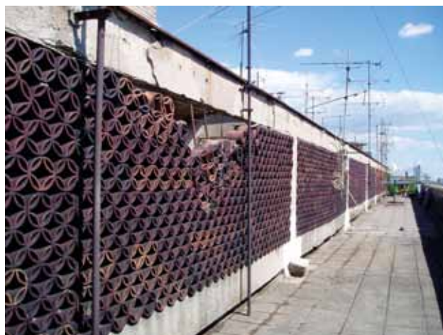
33 Vukovarska 35-35 a, VIII. kat, krovna terasa s ogradom od betonskih prefabrikata (foto: J. Ščavničar Ivković) Vukovarska 35-35 a, 8 th floor, roof terrace with concrete prefabricated railing (photo: J. Ščavničar Ivković)
