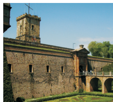
Figure 5. Tower of Montjuïc (Mont-Jouy) Fortress, southern point of the meridian arc (URL8)
