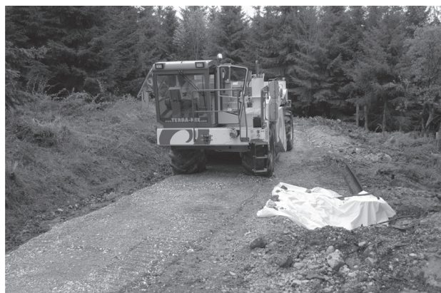
Fig. 2 WR2400 recycler during mixing process
