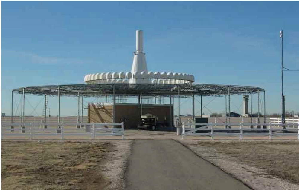
Figure 5. VOR – VHF omnidirectional range with distance measuring equipment
