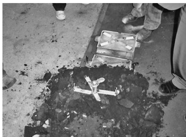
Figure 3 Removal of castings
