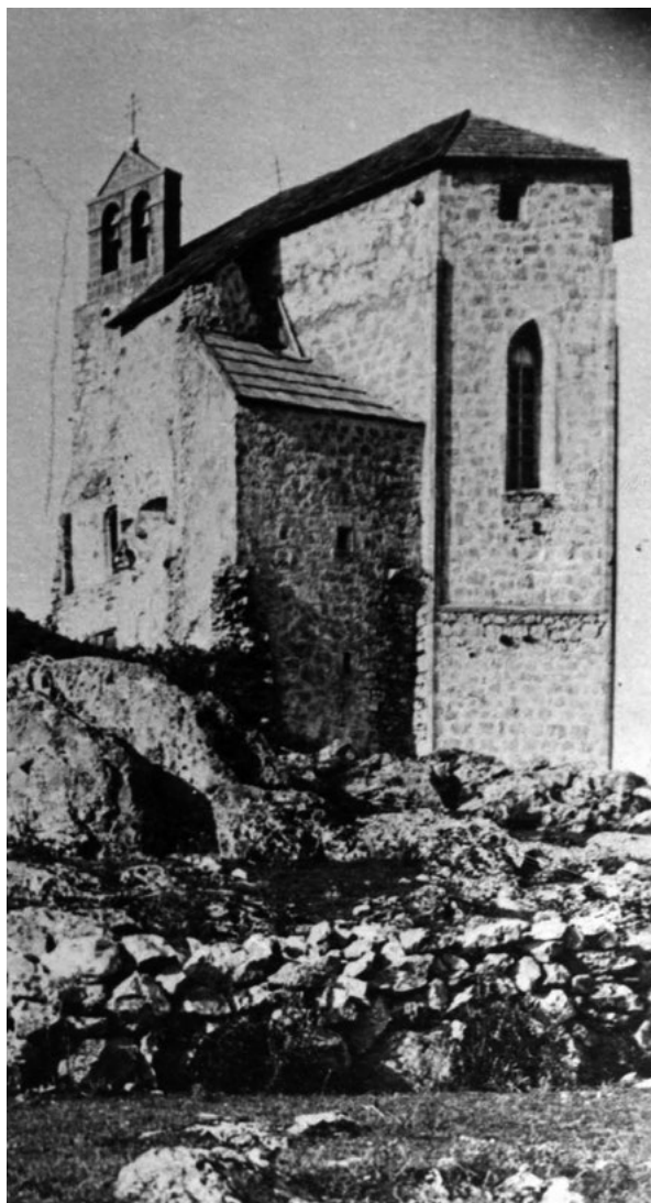
20. Kapela Sv. Trojstva 1917. (fototeka Uprave za zaštitu kulturne baštine Ministarstva kulture, snimio M. Pilar) The Holy Trinity Chapel in 1917 (Photo Archive of the Directorate for the Protection of Cultural Heritage of the Ministry of Culture, photo by M. Pilar)
