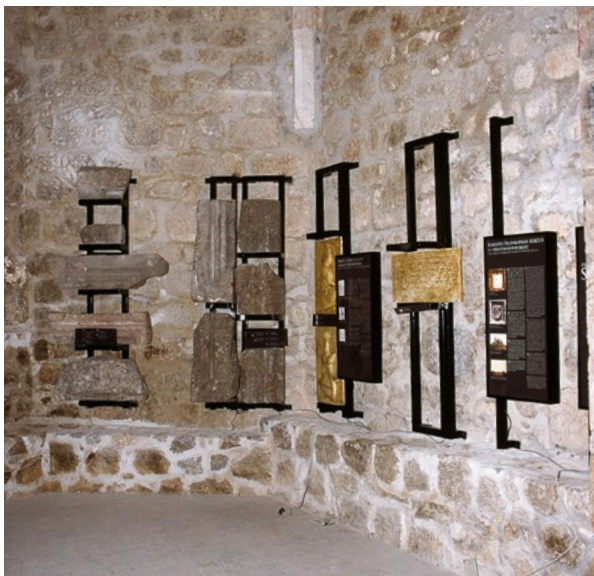
5. Kapela Sv. Trojstva, unutrašnjost substrukcije nakon obnove i postavljanja stalne izložbe (fototeka HRZ-a, snimio D. Miletić) The Holy Trinity Chapel, interior of the substructure after the renovation and setting up the permanent exhibition (Croatian Conservation Institute Photo Archive, photo by D. Miletić)
