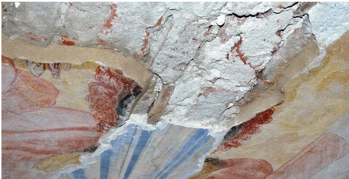
5. Sv. Florijan tijekom konzervatorsko-restauratorskih radova; uklanjanje stare žbukane zakrpe (fototeka HRZ-a, snimila I. Drmić) St. Florian in the course of conservation; removing the old plaster patch (Croatian Conservation Institute Photo Archive, photo by I. Drmić)
