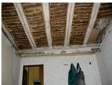
Figure 1 Wooden beams with mud and straw
