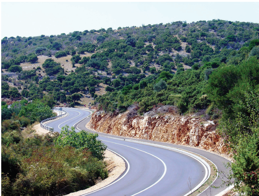
Figure 1: Road cut through the Upper Cretaceous sediments (photo: M. Kovačić, 2008).
