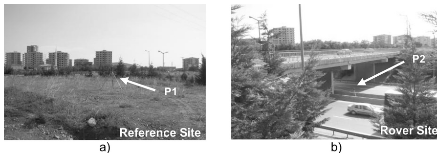
Figure 2 Reference point (P1) and rover point (P2) close to the bridge
