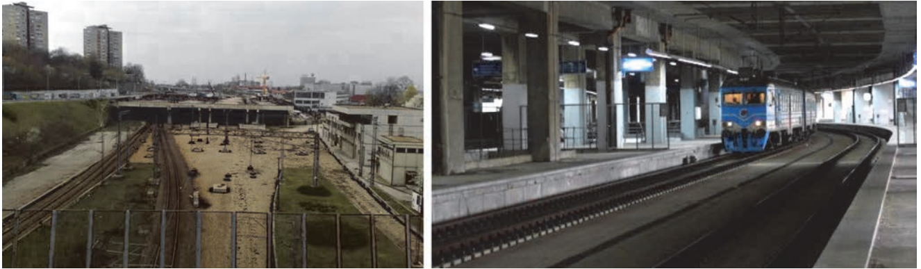
Figure 8. Station at Prokop: a) Nonexistent complex; b) existing railway infrastructure
