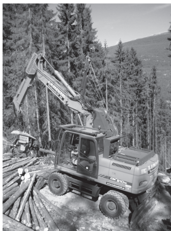
Fig. 2 The Zöggeler yarder at work on the study site
