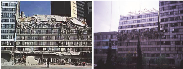
Figure 2 Earthquake in Mexico City, September 19, 1985
