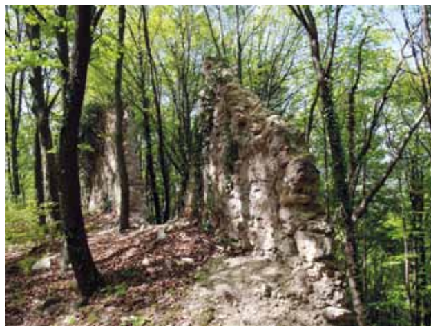
15 Djelomično urušeni sjeverni zid centralnog platoa utvrde Grebengrad, stanje 2009. (foto: M. Korunek) Partially collapsed northern wall of the central plateau of Fort Grebengrad, condition in 2009 (photo: M. Korunek)
