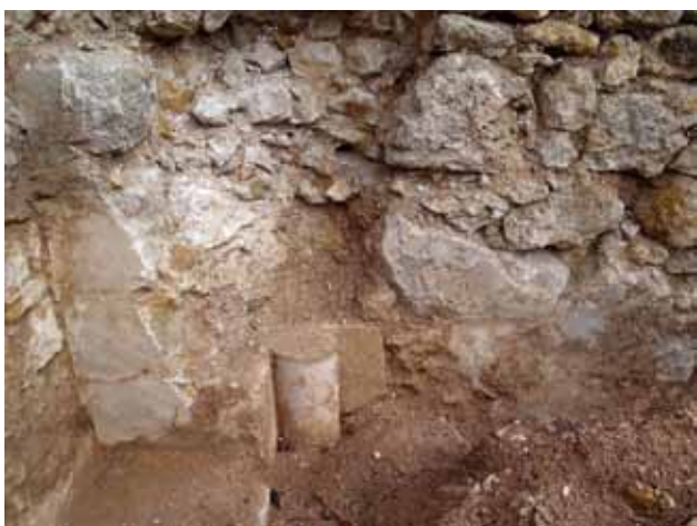
23 Proširenje sjevernog zida lađe, ostatci žbuke i polustup (služba) na spoju sjevernog i istočnog zida kapele utvrde Grebengrad otkriveni tijekom radova 2012. (foto: M. Korunek) Extension of the nave northern wall, remains of plaster and jamb (service) at the junction of the north and east wall of the chapel of Fort Grebengrad discovered in the course of works in 2012 (photo: M. Korunek)
