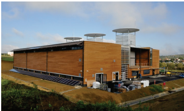
Figure 10 The new RATI Factory building with the 12 kWp PV plant and the Venturi-towers)
