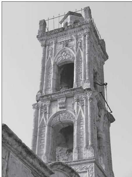
Yet again, the character of the wall surface of the tower indicates a later date of construction, compared to the wall surface of the body of the church.
