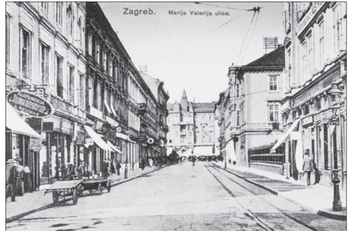
FIG. 5. FRANZ KLEIN & JANKO NIKOLA GRAHOR SENIOR: THREE-STORY CORNER APARTMENT HOUSE SIEBENSCHN, 2 PRERADOVIĆEVA ST, 1873, FRONT FROM PRERADOVIĆEVA (CVJETNI) SQ, RADICALLY REMODELED
