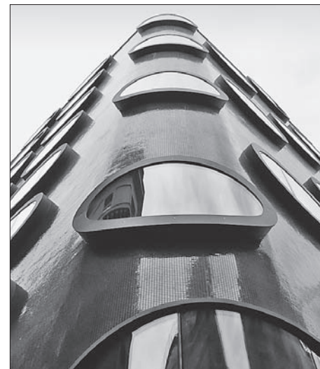
SL 3. HOTEL TOPAZZ, BEČ – DETALJ PROČELJA FIG. 3. HOTEL TOPAZZ, VIENNA – FAÇADE DETAIL
