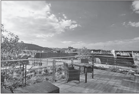
Sl. 10. HOTEL/HOSTEL MOSAIC HOUSE, PRAG – ZELENI KROV I TERASA
