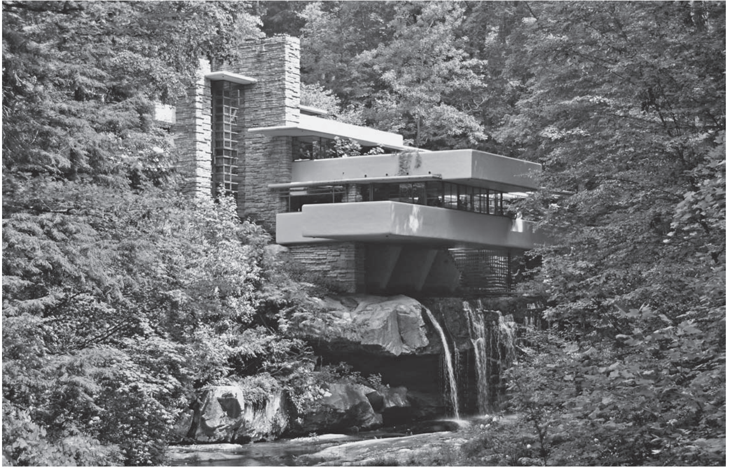
FIG. 1. FRANK LLOYD WRIGHT: FALLINGWATER HOUSE, BEAR RUN, PENNSYLVANIA, 1939. A UNIQUE EXAMPLE OF ORGANIC ARCHITECTURE IS THE KAUFMANN RESIDENCE OR FALLINGWATER HOUSE IN BEAR RUN, PENNSYLVANIA (1935-1939). THE THREE-STORY WEEKEND HOUSE IS SET IN A VERY UNUSUAL LOCATION: ON A CLIFF ABOVE A WATERFALL. THE CANTILEVER STRUCTURE SITS ON TOP OF THE WATERFALL, WHICH IS INVISIBLE BUT CAN BE HEARD. THE HOUSE IS A PRIME EXAMPLE OF A MODERN TECHNOLOGY IN NATURAL SURROUNDINGS.
