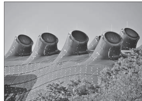
FIG. 13. PETER COOK AND COLIN FOURNIER: GRAZ ART MUSEUM, AUSTRIA, 2003. CONSTRUCTED FROM ABOUT 1,300 INDIVIDUALLY SHAPED, TRANSLUCENT PLEXIGLAS PANELS COVERING THE BIOMORPHIC BUILDING.
