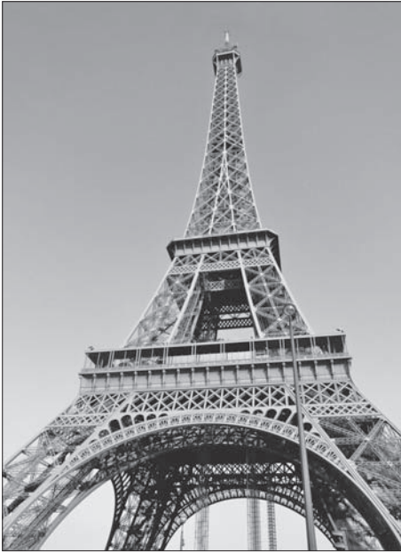
FIG. 6. GUSTAVE EIFFEL: EIFFEL TOWER, PARIS, FRANCE, 1889. CONSTRUCTION WAS INSPIRED BY THE HUMAN FEMUR BONE, WHICH IS VERY GOOD AT HANDLING OFF-CENTRE STRESSES.
