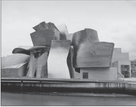
FIG. 11. FRANK GEHRY: GUGGENHEIM MUSEUM, BILBAO, SPAIN, 1997. THE MUSEUM, ALTHOUGH HEAVILY DEPENDENT ON DIGITAL CURVED SURFACE MODELLING SOFTWARE, WAS DEVELOPED FROM SUCH GESTURAL AND SENSUAL INVESTIGATIONS IN SKETCH AND MODEL FORM. ONCE THE SCULPTED FORM WAS FINALIZED, AN EXACT DIGITAL MODEL DESCRIBED THE BUILDING IN MATHEMATICALLY DEFINED CURVES AND SURFACES.
