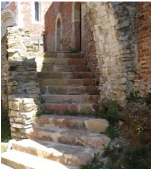
9. Kameno stubište prema kapeli s crvenim tragovima vatre (snimio H. Malinar). Stone staircase leading to the chapel with red traces of fire (photo by H. Malinar)
